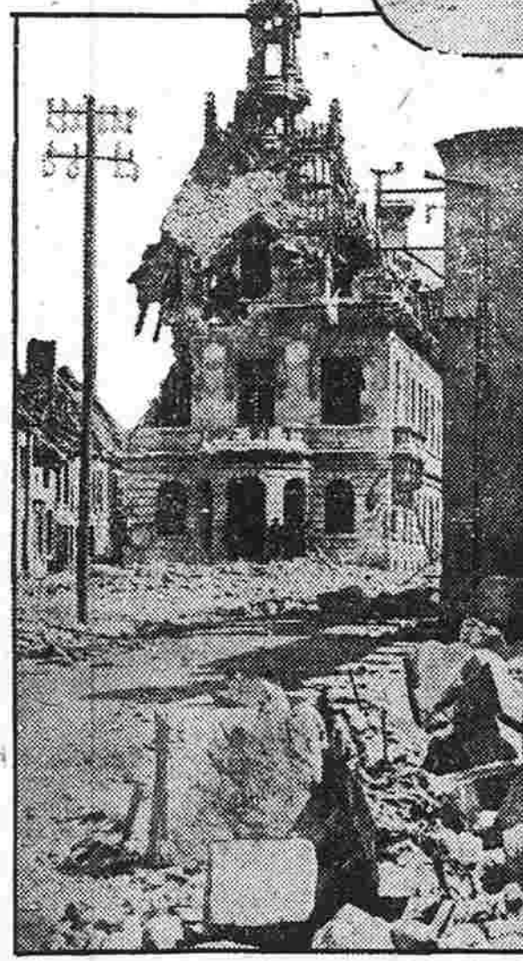
Fismes city hall . . . suffered heavy bombardment from both sides in the struggle of August, 1918.
